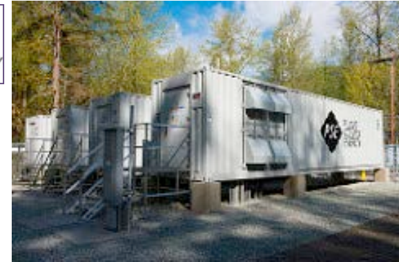
2 MW/4.4 MWh lithium-ion/phosphate battery Glacier, WA
